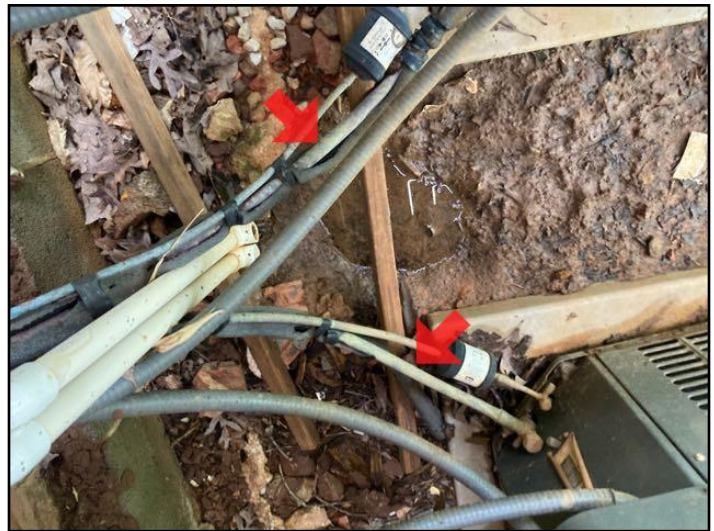
96. Insulation missing
