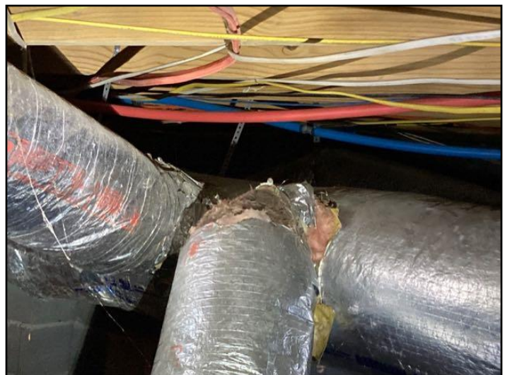
89. Damaged insulation
