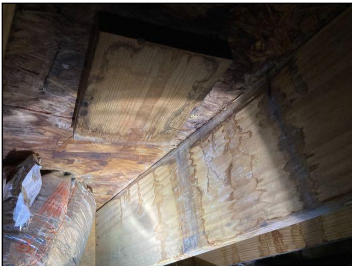
70. Patch repair under living/kitchen area
