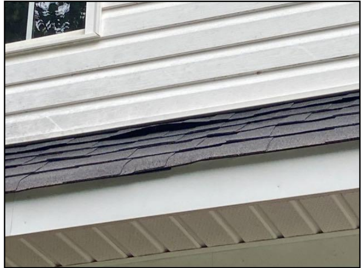
8. Shingle or flashing uplift
