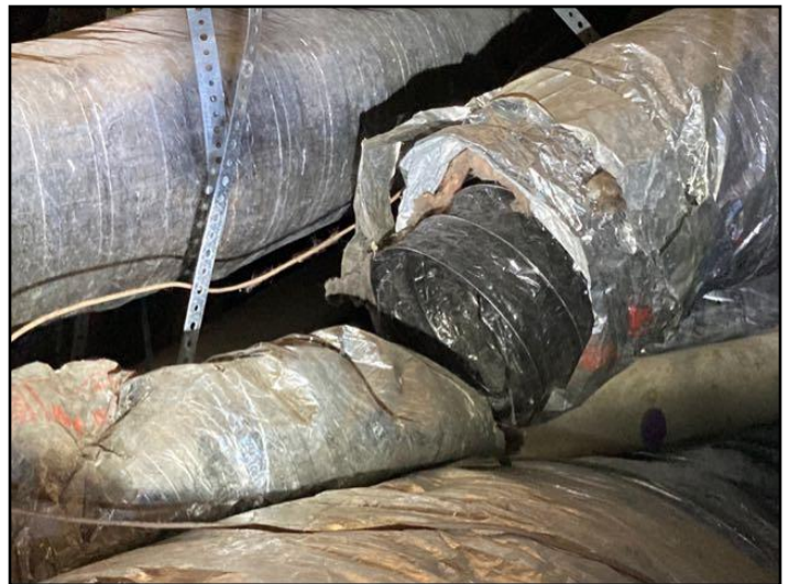
85. Disconnected duct
