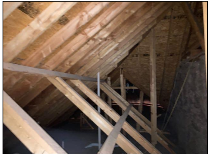
61. Rafters/ceiling joists
