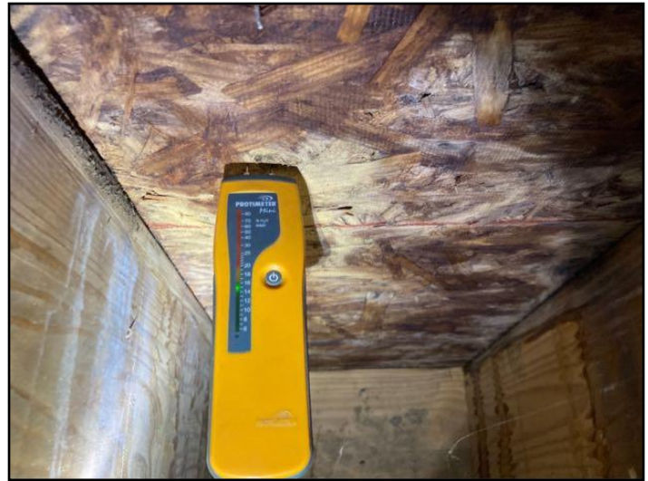
69. Acceptable moisture content under kitchen
