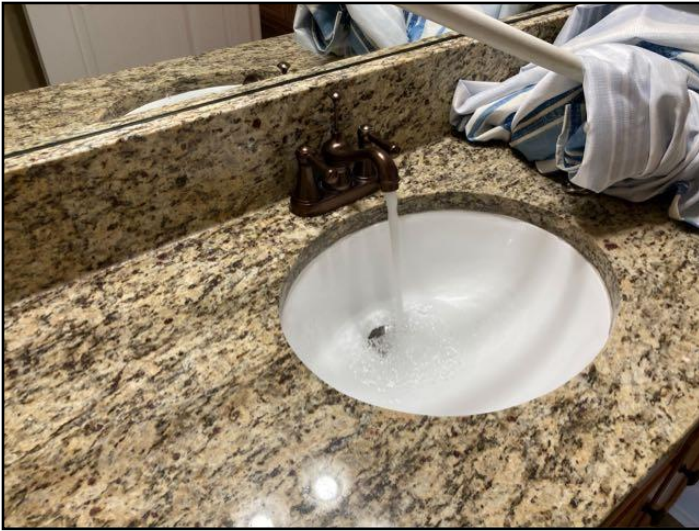
127. Sink is functional
