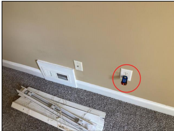
76. Reversed polarity
