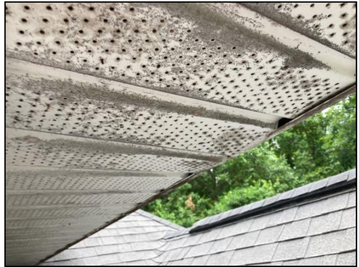
17. Soffit popped out of place
