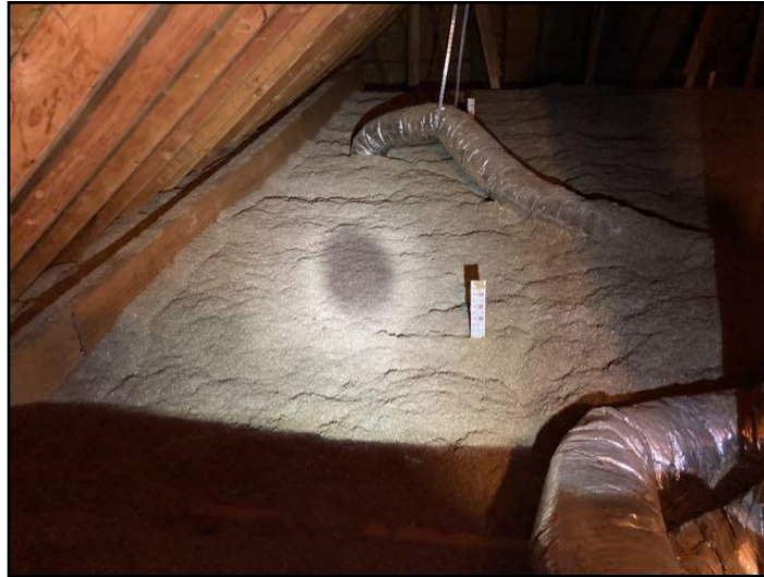
105. View of insulation
