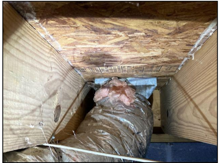
87. Damaged insulation
