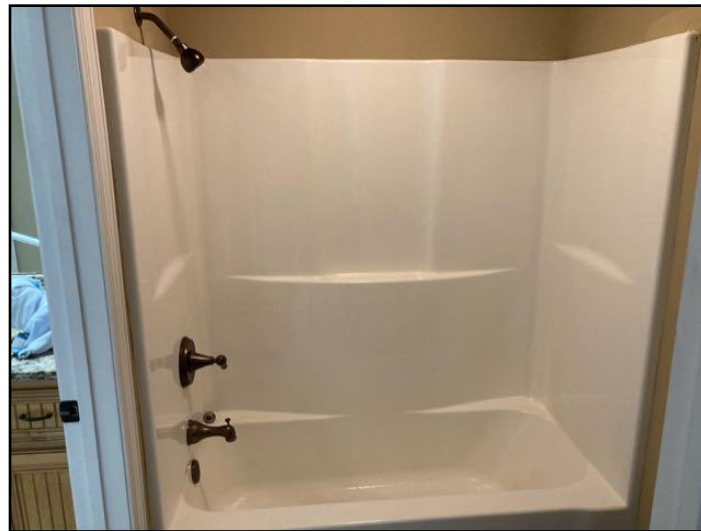
136. Tub/shower is functional
