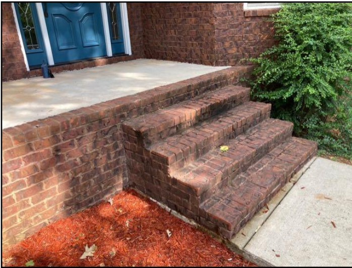
47. Handrail missing
