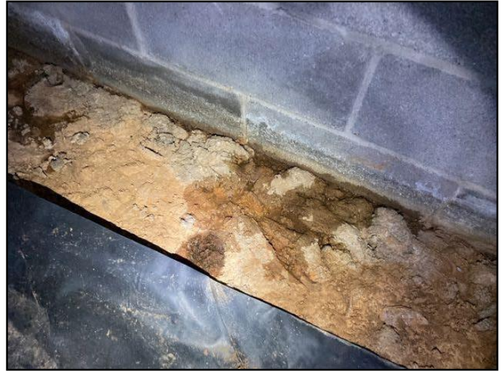
57. Water seepage at left side
