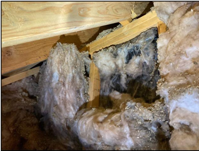
106. Damaged insulation
