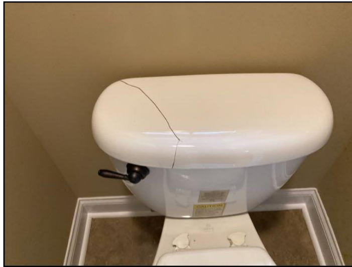
137. Cracked tank lid
