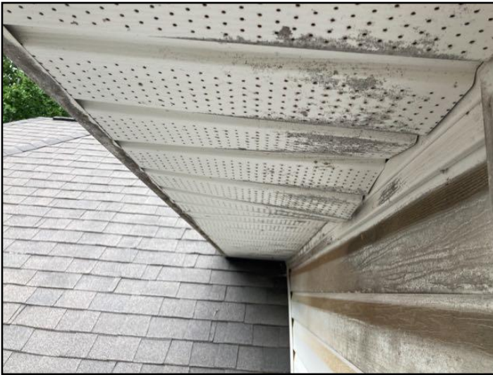
16. Soffit popped out of place
