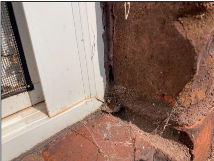
19. Caulking/mortar gap
