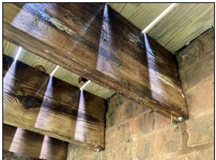
31. Deck joist connection detail
