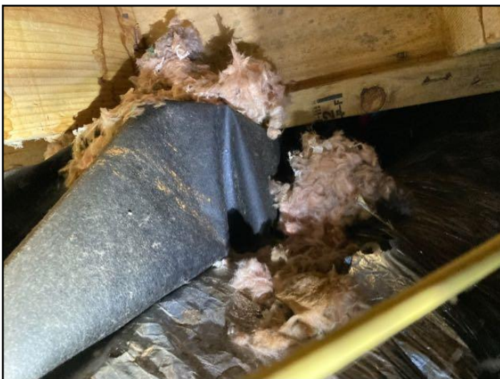
88. Damaged insulation
