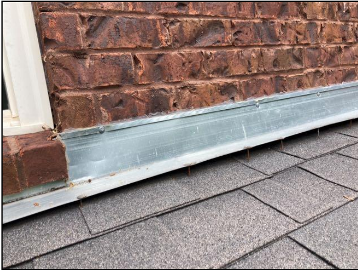
7. Flashing uplift
