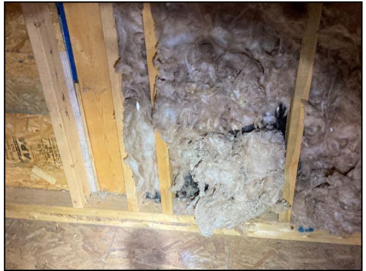
107. Damaged insulation
