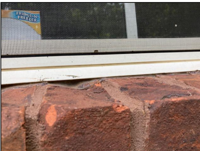
21. Caulking/mortar gap
